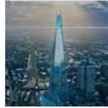
The Shard London Bridge Tower London, UK
